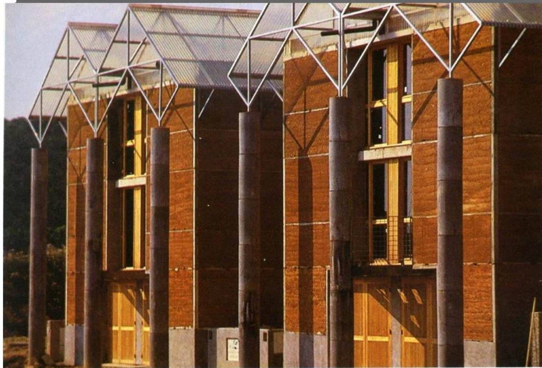
BUILDING NEAR GRENOBLE (FRANCE). PROJECT OF THE 80s IN WHICH 64 HOUSING UNITS BUILT WITH DIFFERENT TYPES OF CONSTRUCTION TECHNIQUES WITH LAND WERE BUILT. SOURCE: ARCHITECTURES DE TERRE
