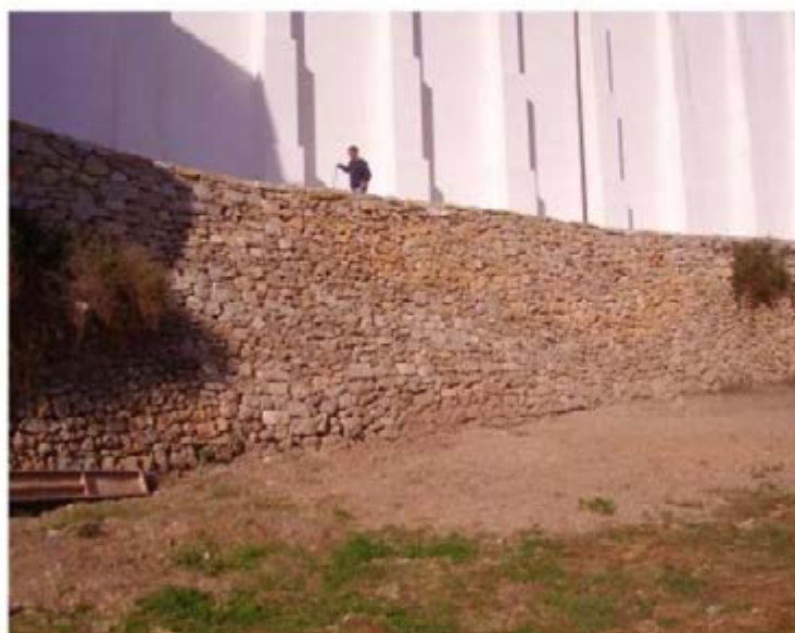
Retaining wall of a street
